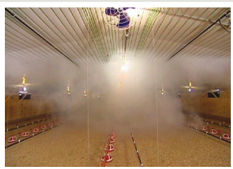
DirectAire Inlets direct air along ceiling towards center of poultry house
